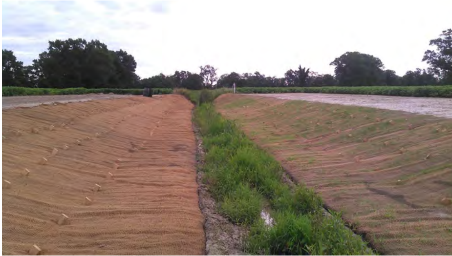
Figure 10. Two-stage ditch example showing the extended benches within the ditch. This two-stage ditch is located in Talbot County, MD
