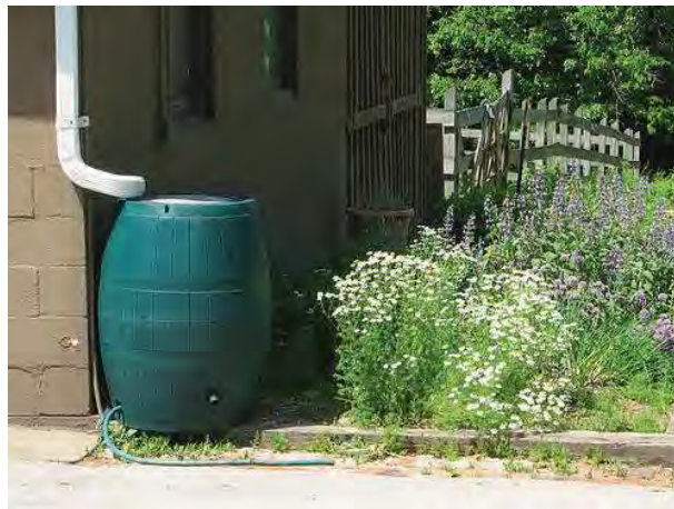
Figure 6. Example of a downspout disconnected from the driveway and redirected to a rain barrel. Downspout disconnections can also be redirected to lawn or other vegetated spaces rather than into a barrel.
