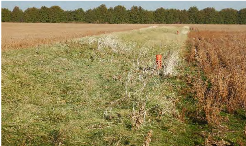
Figure 12. This photo depicts a WASCOB with a berm running across a grassed drainage area and two orange risers that help convey stormwater in a less erosive manner. Photo from Essex Soil and Crop Improvement Association, http://escia.ca/2019-conservation-farm-award/wascob/
