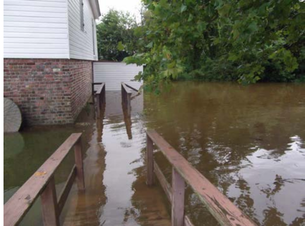
Figure 34. Flooding of the Old Wye Mill during a storm event in 2017. Photo from The Old Wye Mill Facebook page.
