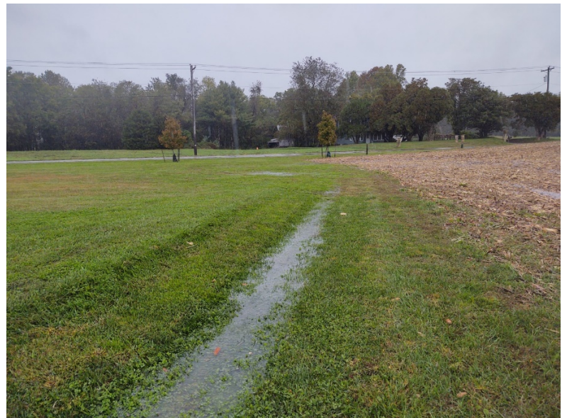
Figure 27. This bioretention would receive water from an existing grassed swale that collects water from the Nagel Grain facility. The bioretention could potentially be designed to intercept water from the adjacent farm field. The outlet of the bioretention would need to go under Route 404 in a pipe with an outlet into the proposed wetland area. The bioretention to the west of this site could be tied into this bioretention if elevations permit.
