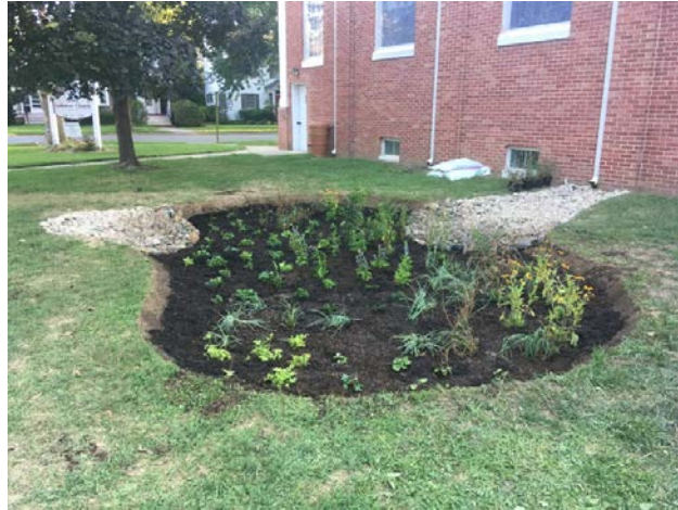
Figure 9. Bioretention project at a church in Easton, MD.
