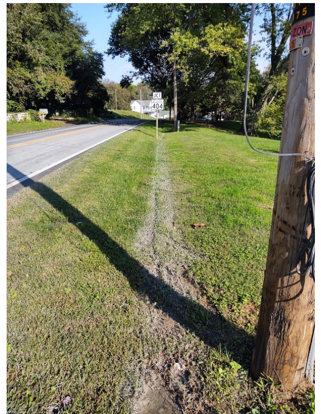
Figure 32. The current roadside ditch is shallow and in need of repair. There are multiple culverts for each driveway that in some instances are blocked. The ditch abruptly ends at the intersection of Old Wye Mills Rd. and Route 404, causing sheet flow across the roads during storm events. This ditch enhancement would reshape the ditch so that it can convey water in a less problematic manner, help better infiltrate water to reduce stormwater volume, and add a stormwater drain at the end so water does not sheet flow across the road.
