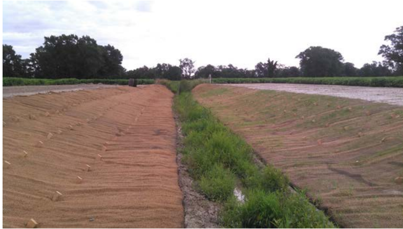
Figure 22. Two-stage ditch example showing the extended benches within the ditch. This two-stage ditch is located in Talbot County, MD.
