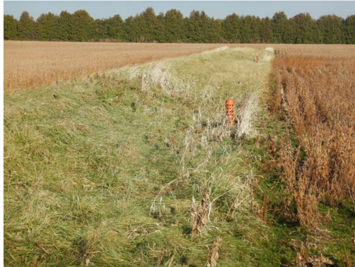
Figure 24. This photo depicts a WASCOB with a berm running across a grassed drainage area and two orange risers that help convey stormwater in a less erosive manner. Photo from Essex Soil and Crop Improvement Association, http://escia.ca/2019-conservation-farm-award/wascob/
