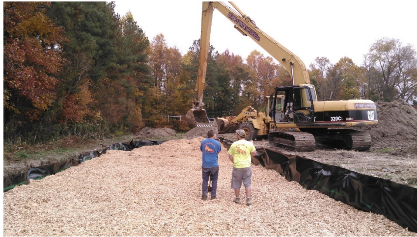
Figure 17. Denitrification Bioreactor example showing the subsurface woodchip-filled pit.
