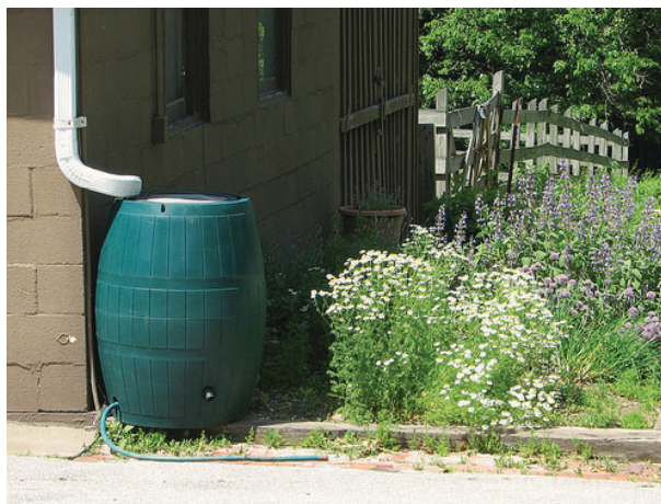
Figure 14. Example of a downspout disconnected from the driveway and redirected to a rain barrel. Downspout disconnections can also be redirected to lawn or other vegetated spaces rather than into a barrel.
