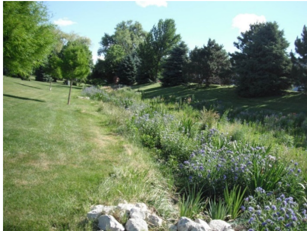
Figure 11. Example of a vegetated open swale in Maryland.
